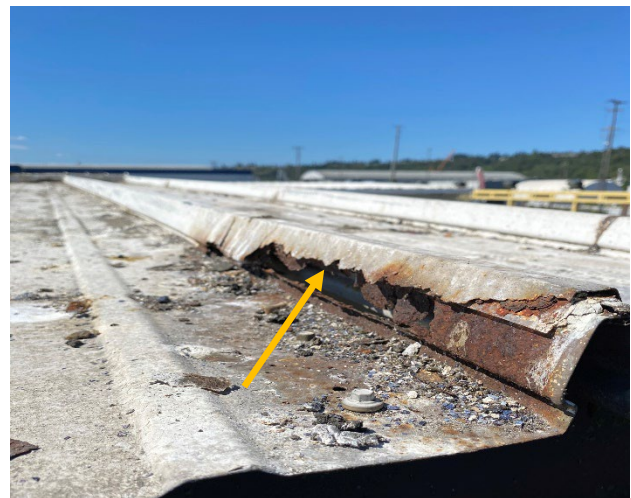
Exhibit E – Corrosion at Existing Roof Panel
