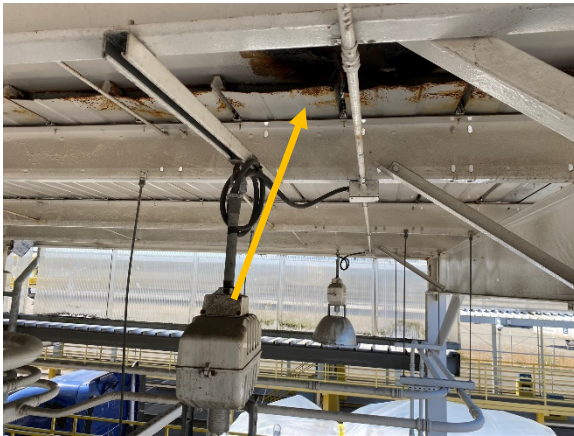
Exhibit B – Deterioration at Underside of Panel
