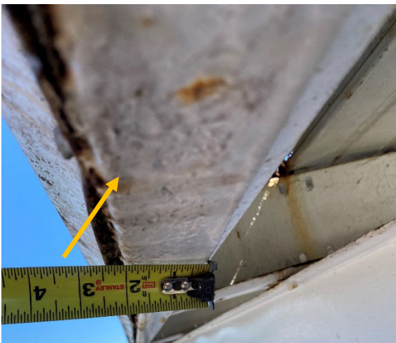
Exhibit D – Corrosion at Structural End Channel
