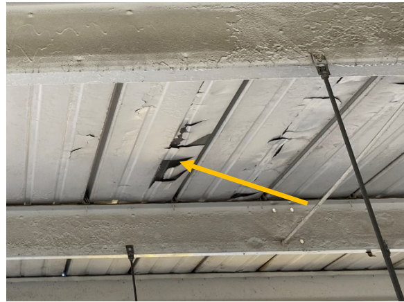
Exhibit C – Flaking and Exposed Panel Substrate
