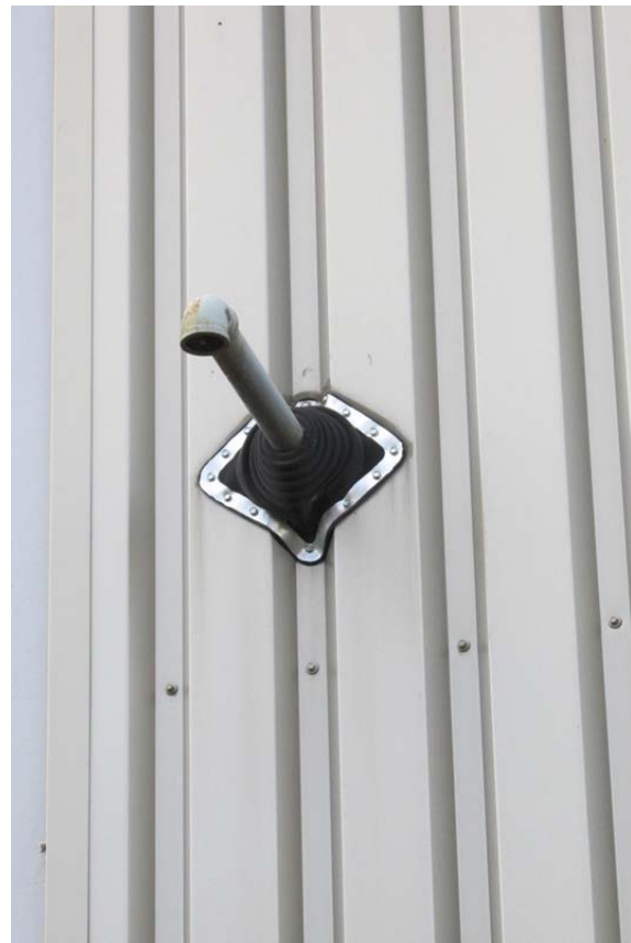
Figure 12 Boot flashing at vent pipe
