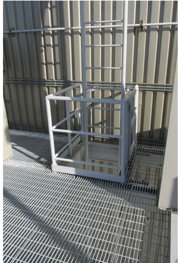
Figure 23 Ladder & Opening in Mech. Mezzanine Floor
