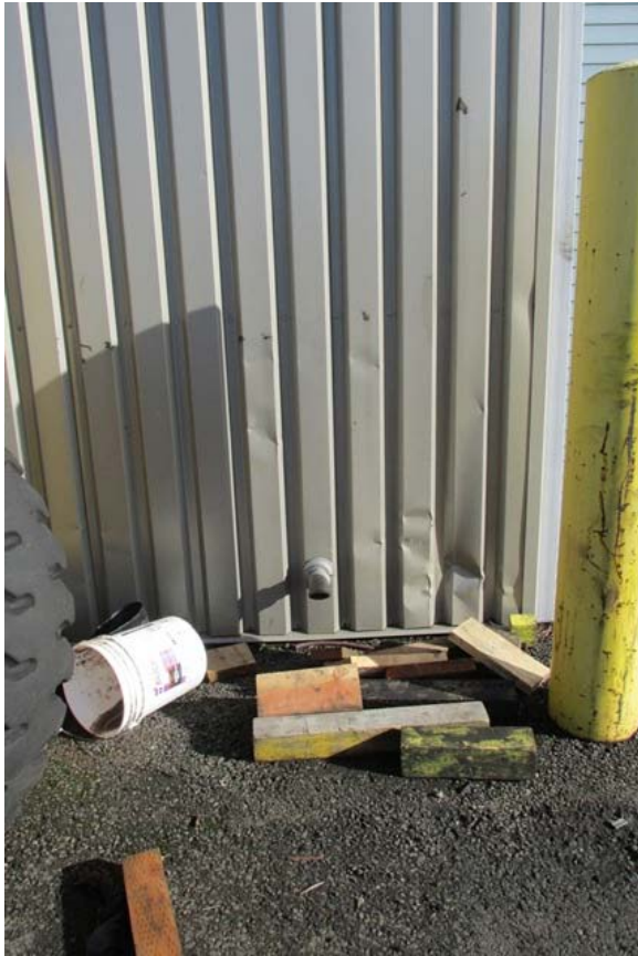
Figure 14 Damage to base of wall at north end of building
