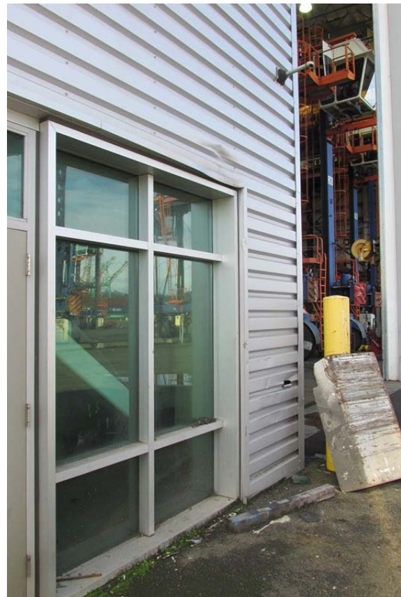
Figure 6 East Elevation, base of Tower at metal wall panel damage
