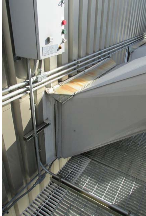
Figure 26 Mech. Mezz. Duct penetration of West wall.
