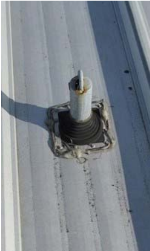
Figure 28 Typical Fall Restraint Stanchion
