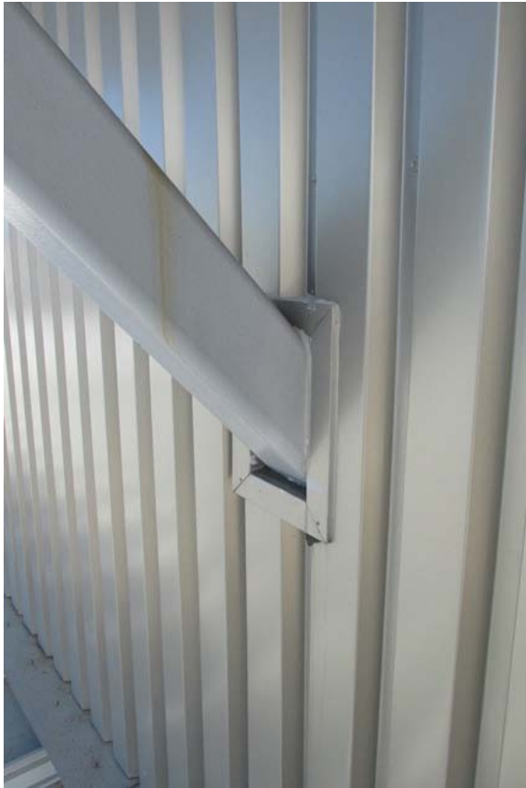
Figure 31 Wall penetration at Mech. Mezz support brace.
