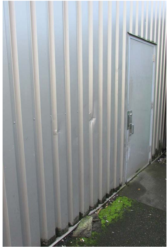
Figure 9 East Elevation, wall damage at northern end of building
