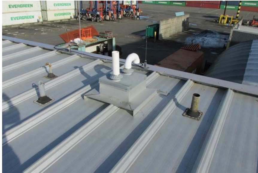
Figure 33 Roof Penetration over Service Bays North end of building view east.
