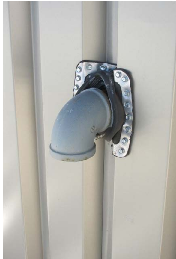
Figure 35 Wall Penetration boot condition.
