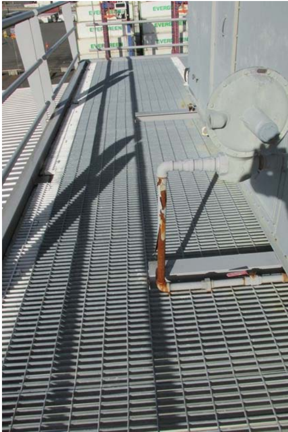
Figure 25 Mech. Mezz. Floor grating and pipe condition.
