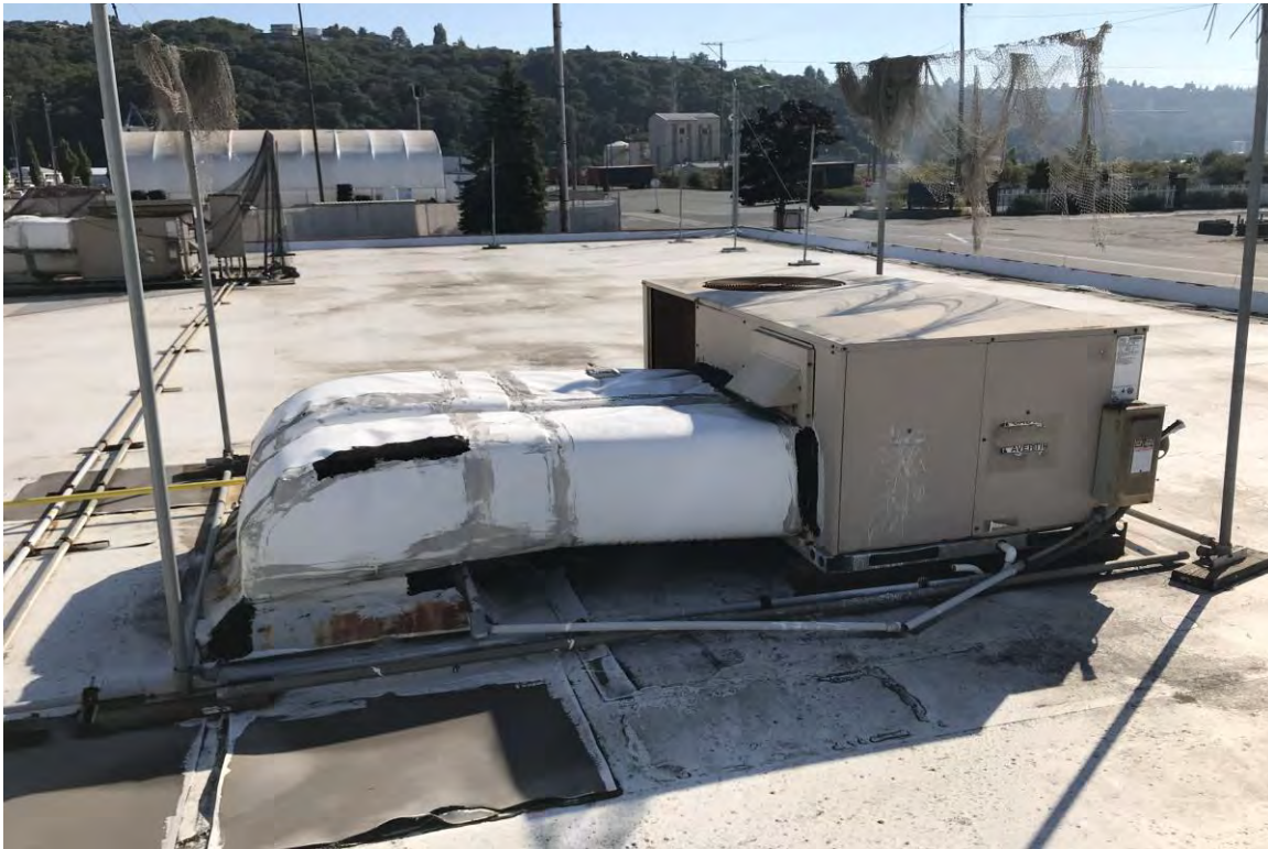
Photograph 3: HVAC system with fiberglass insulation on ducts.
