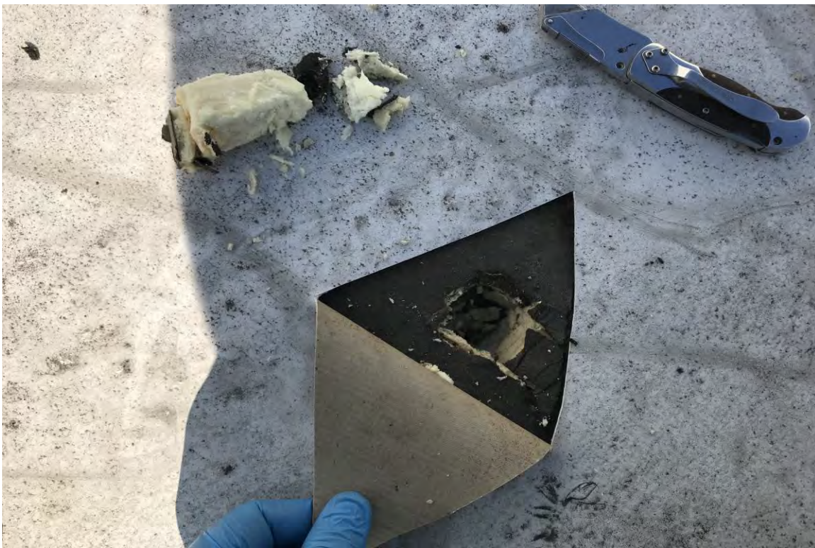
Photograph 4: Typical roof system, no ACM present.
