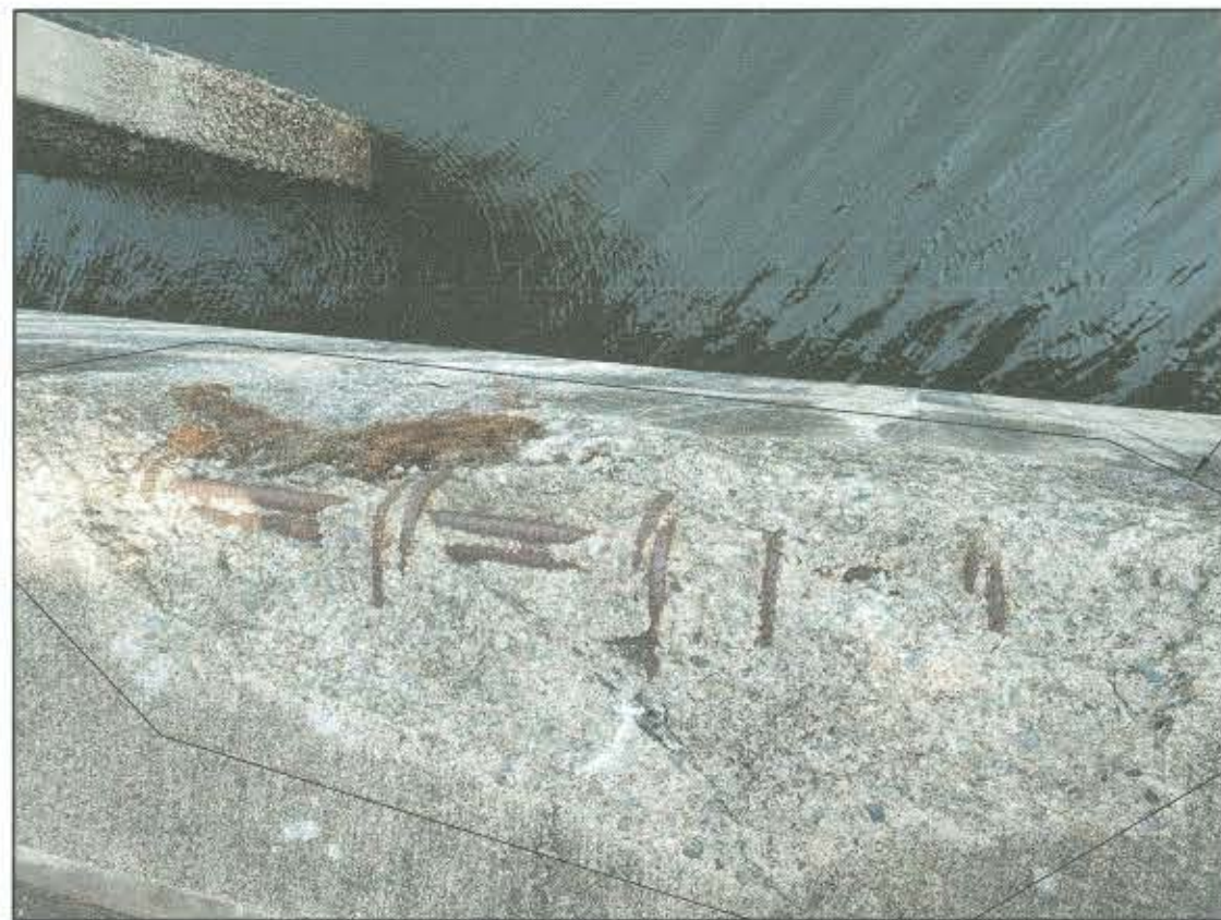
2 BULLRAIL DAMAGE REPAIR PHOTO SCALE: NTS
