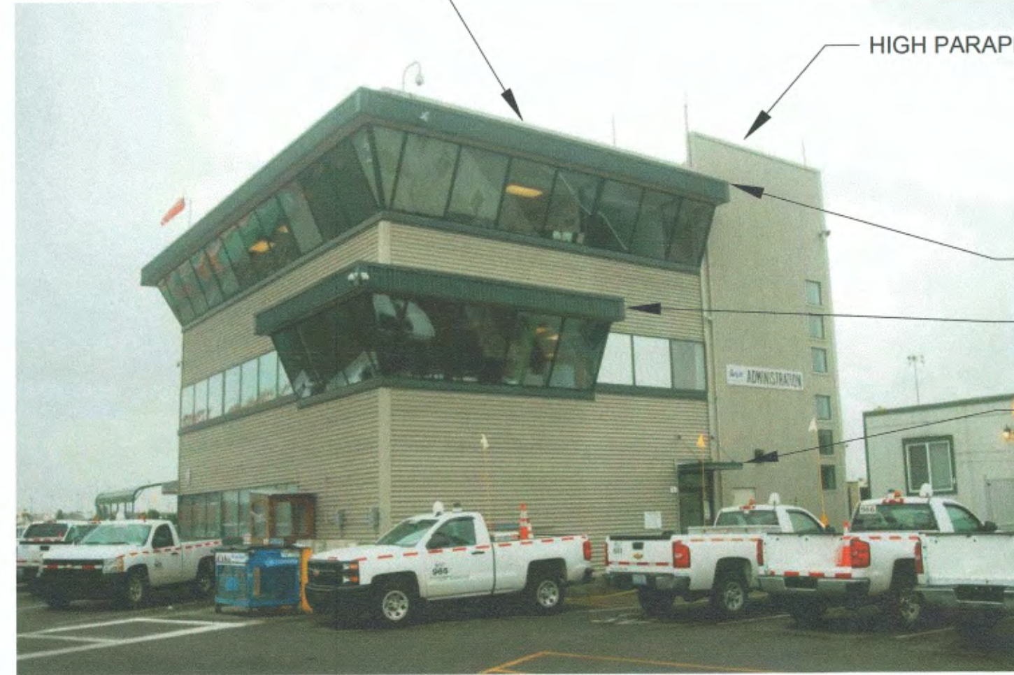
1 ADMINISTRATION BUILDING EXTERIOR VIEW NTS
