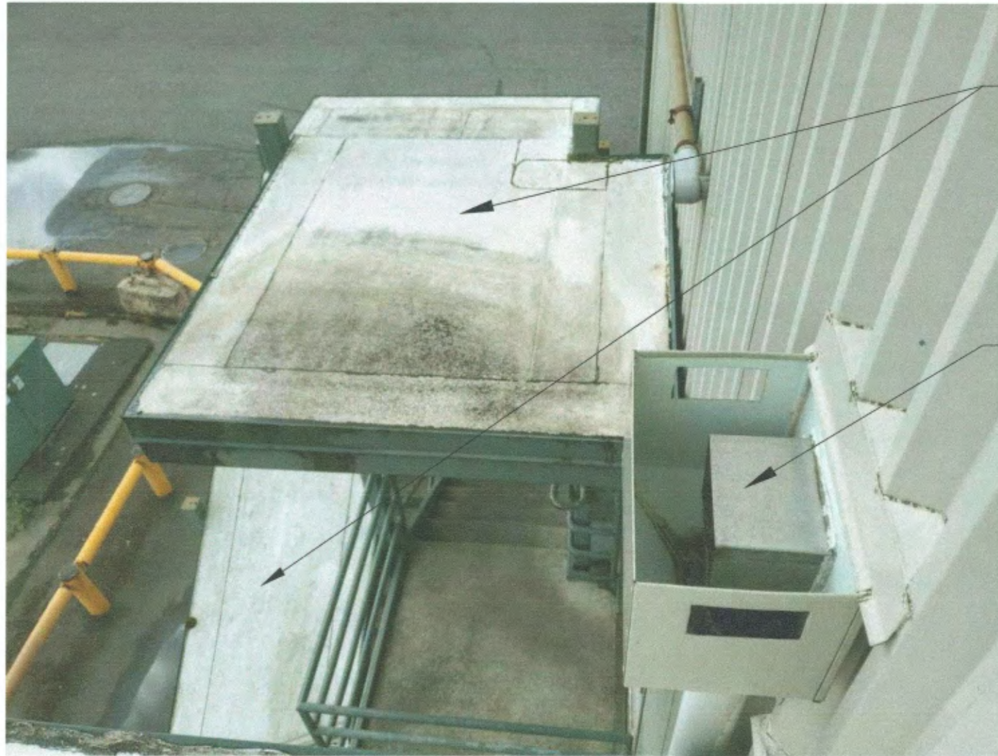
9 NTS ROOF AT STAIR
