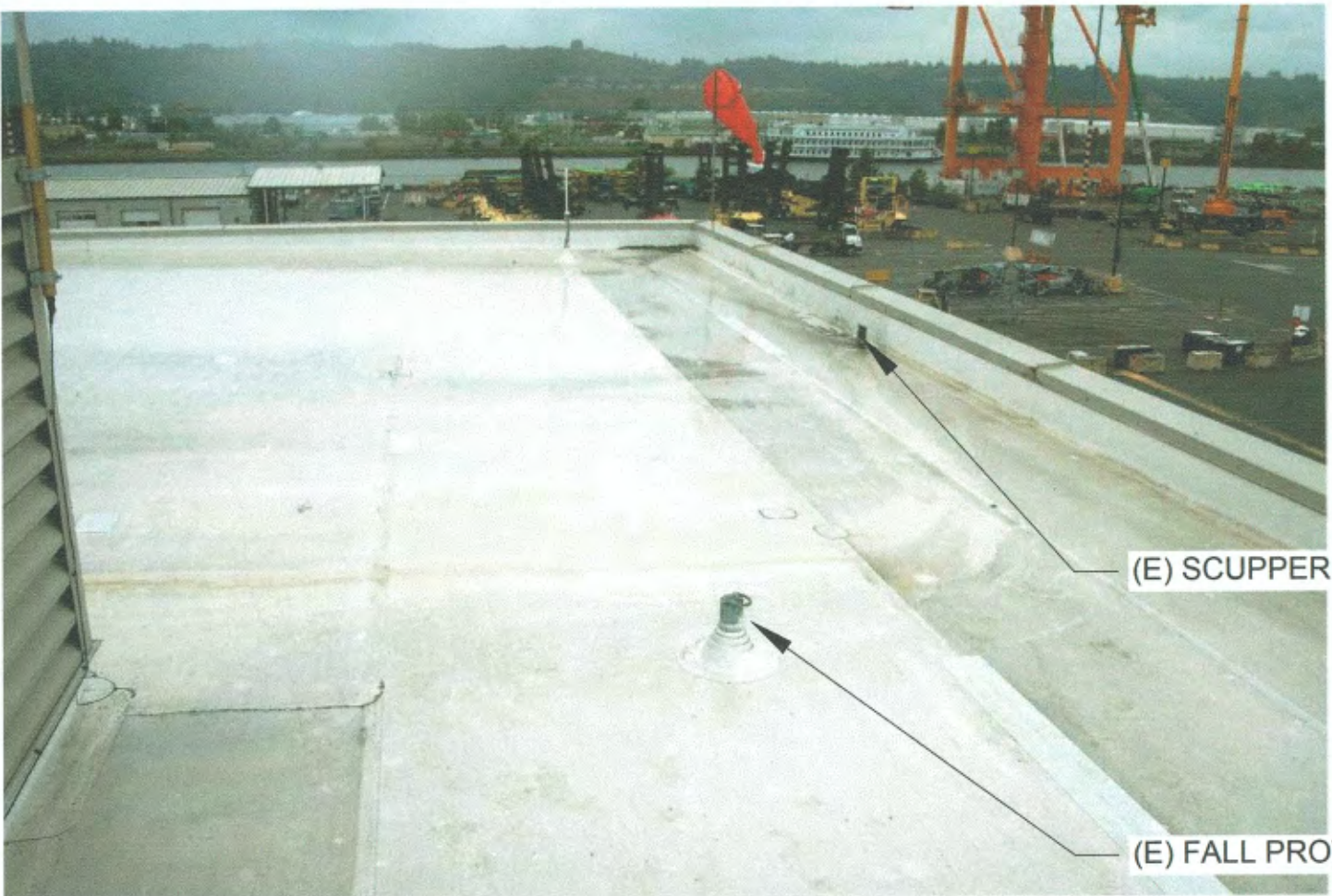
8 LOW PARAPET WALL NTS
