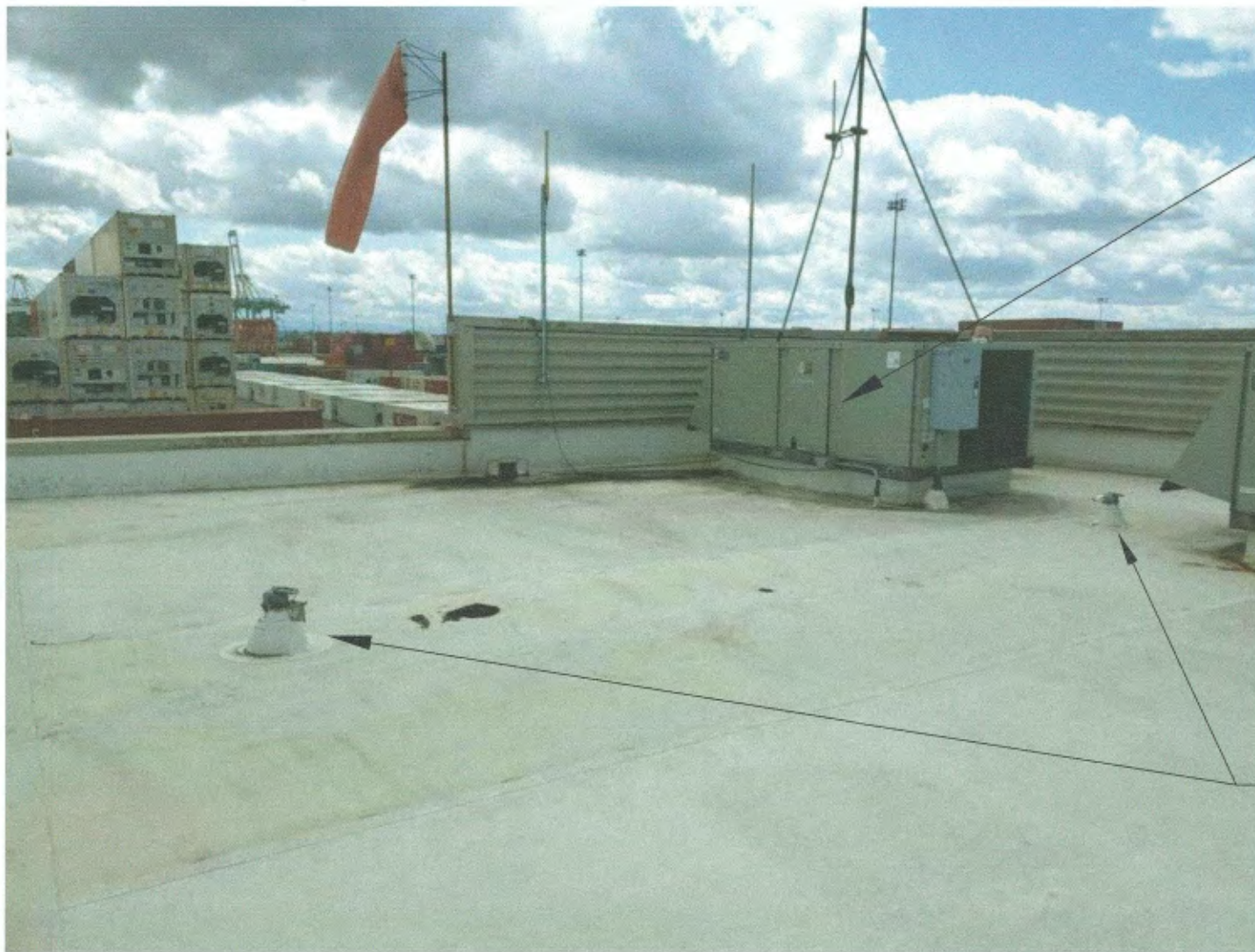
6 NTS (E) ROOF TOP UNIT
