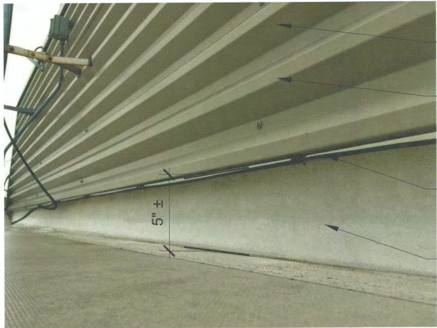
7 BASE FLASHING NTS
