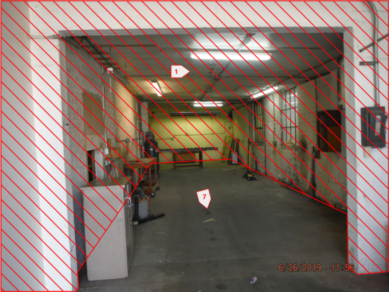
Figure 13 – 2338 E 11 th Street Building Demolition Interior Photograph
