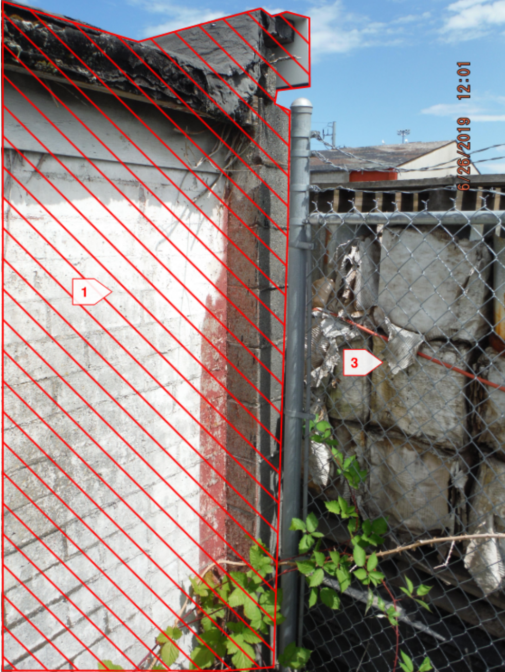
Figure 9 – 2338 E 11 th Street Building Demolition Exterior Photograph
