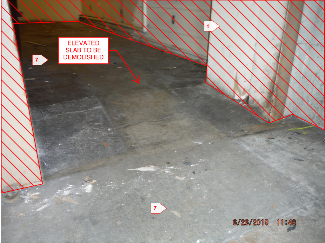
Figure 14 – 2338 E 11 th Street Building Demolition Interior Photograph
