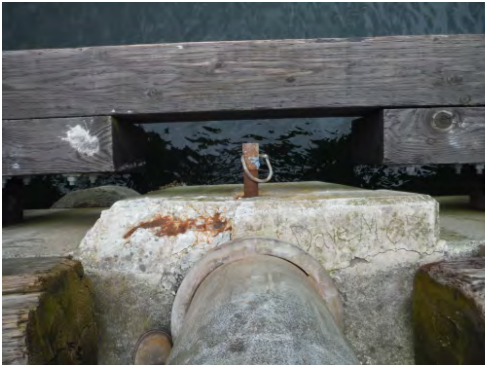
Terminal 7 (Berths A, B, & C) Photo 4 – Typical Pipe Bollard
