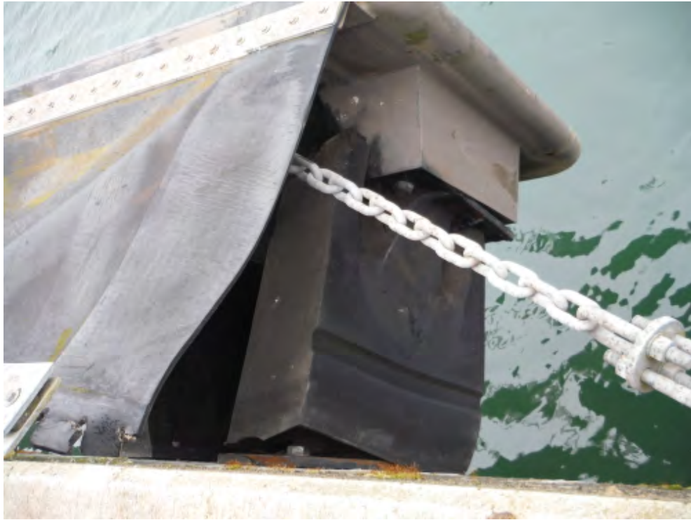
Pierce County Terminal Wharf Photo 3 – Typical Damaged Rubber Fender
