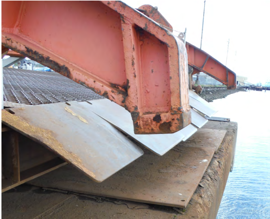
Totem Ocean Trailer Express Photo 1 – Concrete Edge Spalling at Aft Pier
