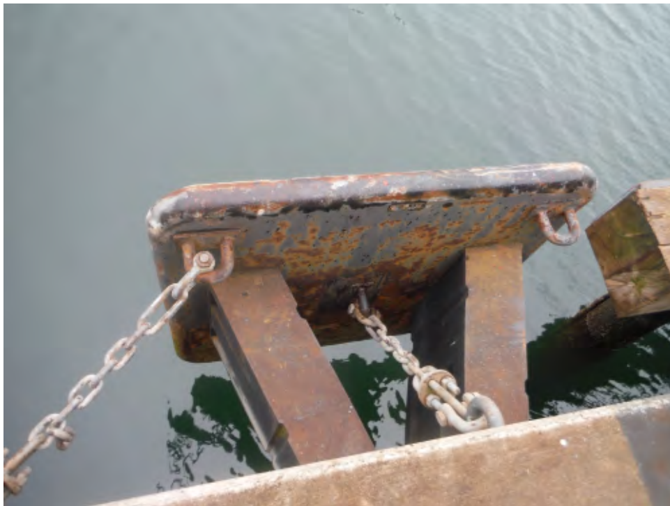
APM Terminal Wharf Photo 3 – Typical Fender Panel
