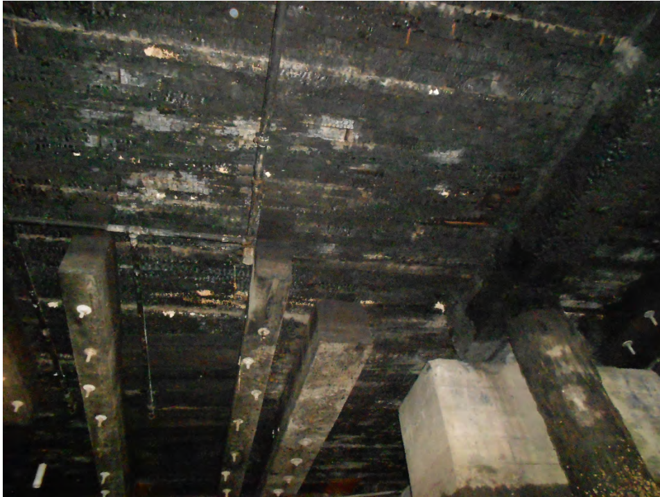
Terminal 7 (Berths A, B, & C) Photo 3 – Typical Charred Timber
