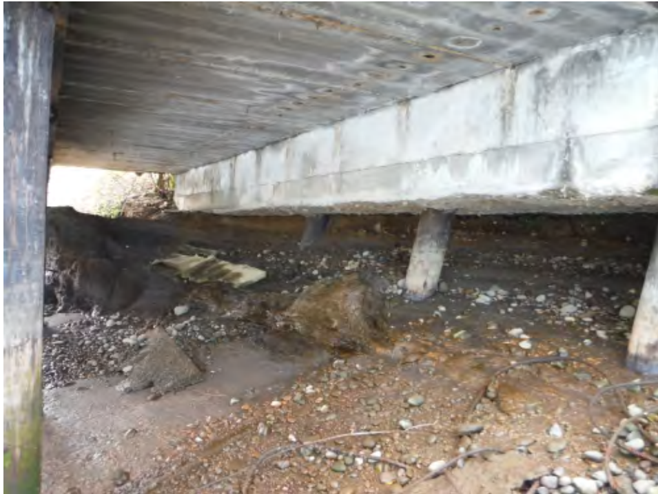
Pony Lumber Dock Photo 3 – Typical Undermining at Bulkhead
