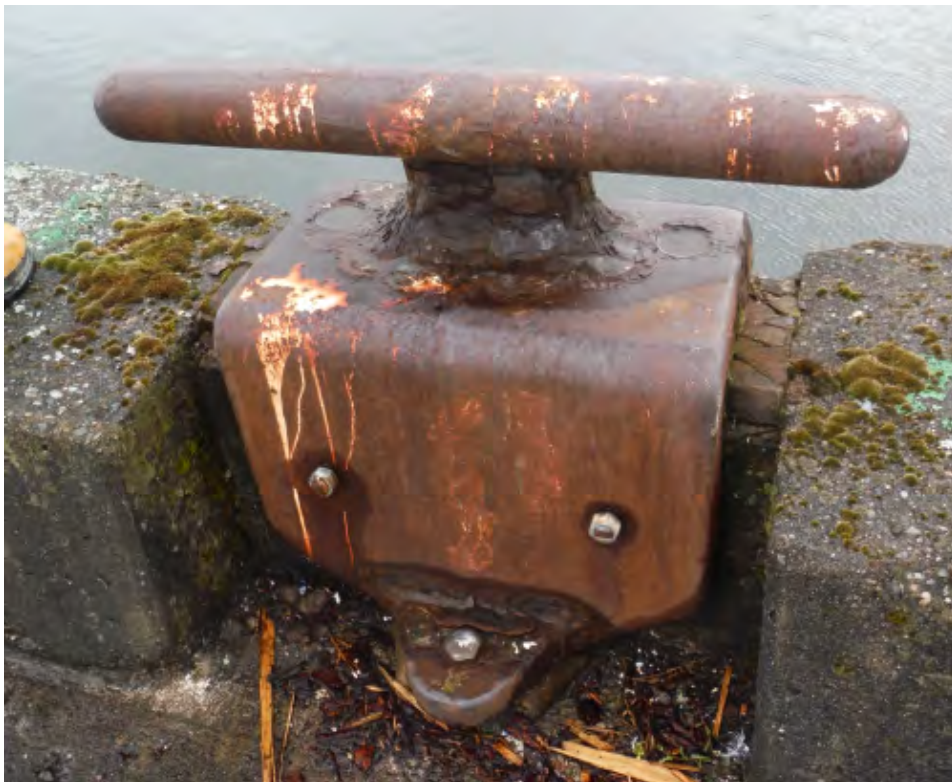
West Hylebos Log Dock Photo 4 – Typical Condition of Mooring Hardware
