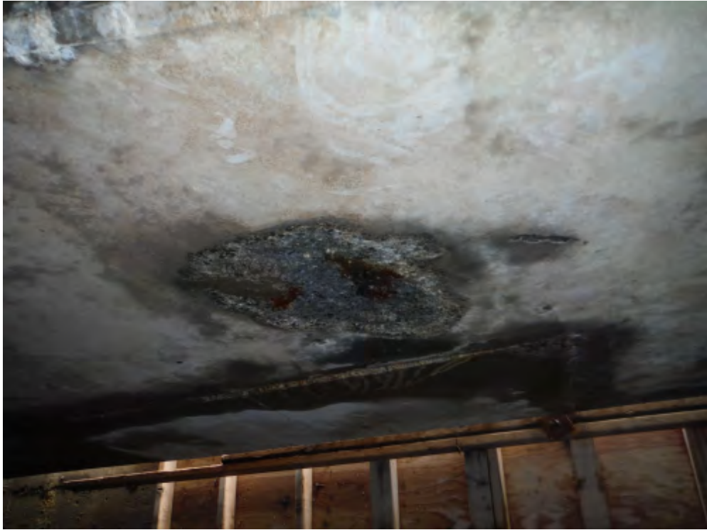
Terminal 4 Wharf (Remaining) Photo 1 – Spall on Deck Panel Soffit Adjacent to New Construction
