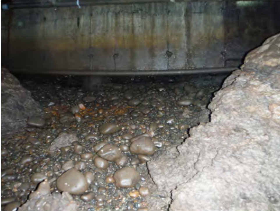
West Hylebos Log Dock Photo 3 – Undermining at Concrete Bulkhead
