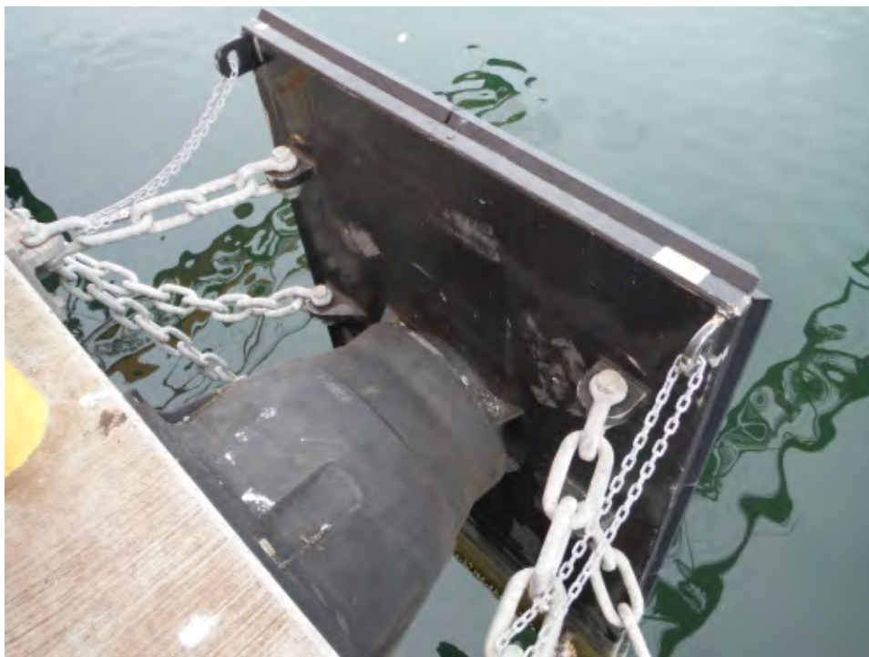
Washington United Terminal Wharf Photo 3 – Typical Fender Panel
