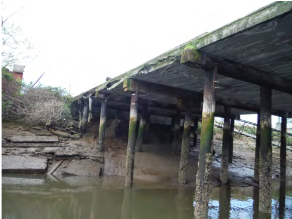
Pony Lumber Dock Photo 2 – Typical Below-Deck Conditions
