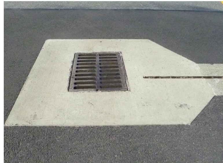
P05 TYPICAL TYPE 1L CB WITH TRENCH DRAIN — NO SCLAE
