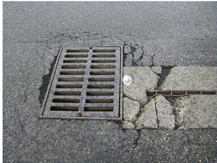
P05 TYPICAL TYPE 1L CB WITH TRENCH DRAIN — NO SCLAE
