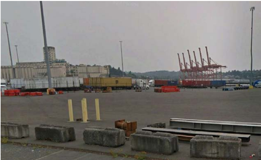
STREET VIEW TERMINAL 10 LOOKING SW
