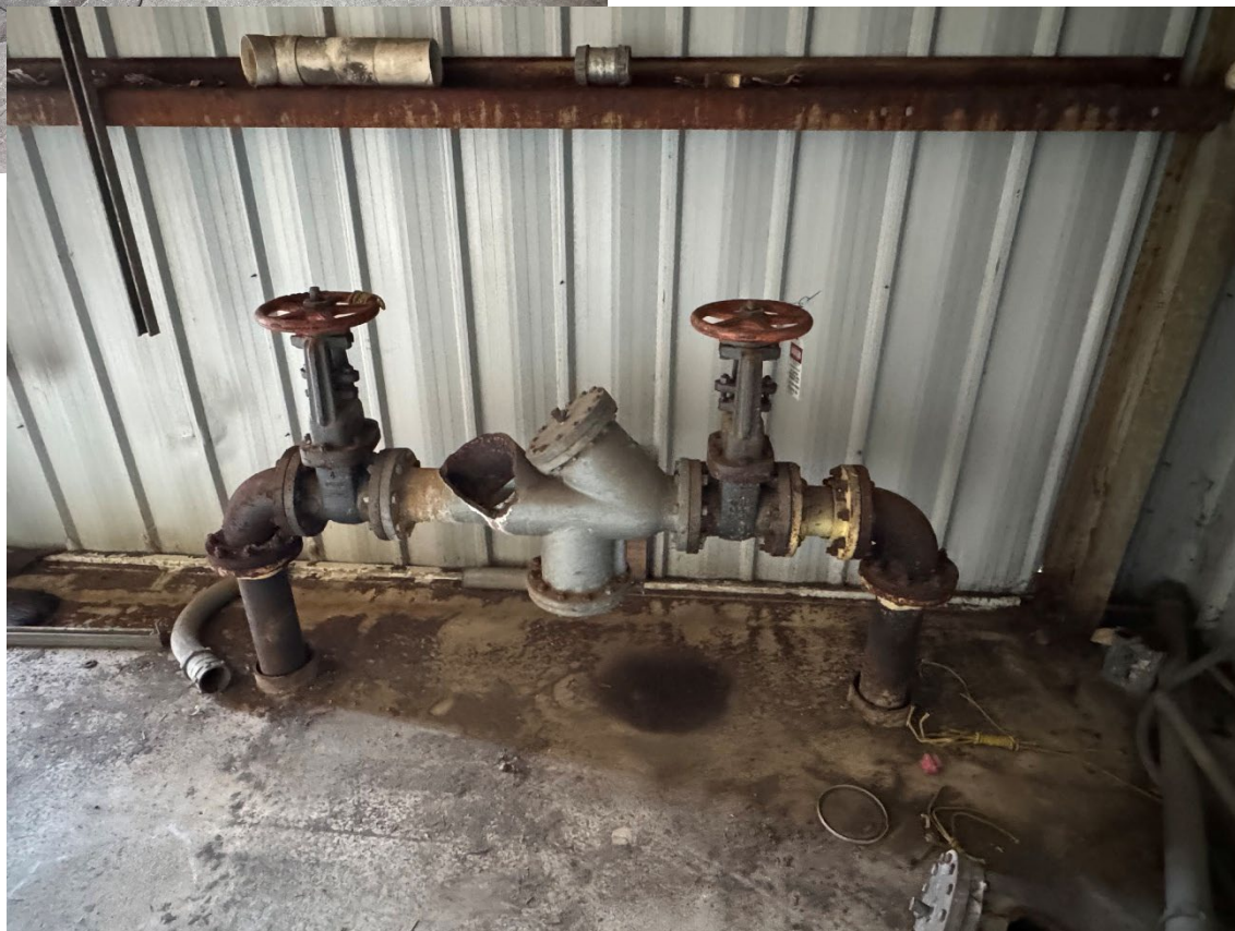
Photo 6 – Pipe riser inside Shed, with AACM gaskets in pipe flanges, and AACM packing inside screw valves. Demolition is planned to slab on grade, which means that this riser would be cut off at concrete. A certified asbestos contractor could cut the riser in-tact, wrap in two layers of 6-mil poly, and dispose as ACM. Other removal methods are also possible.
