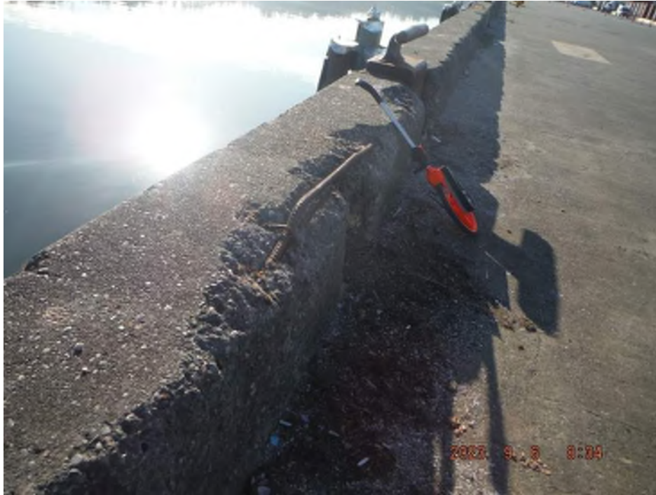
Photo 3 – Concrete Bullrail Mechanical Spall with Deformed Bar at Bent 25.
