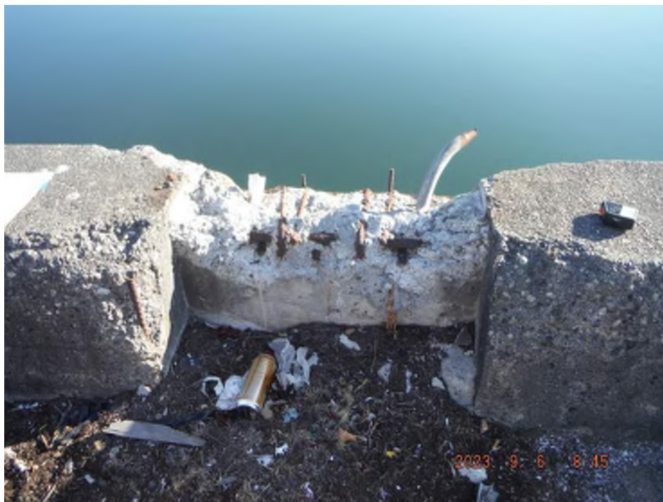
Photo 6 – Missing Cleat at Bent 43.
