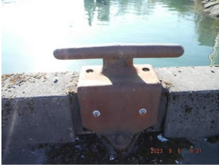
Photo 4. Typical Cleat Mooring Fitting
