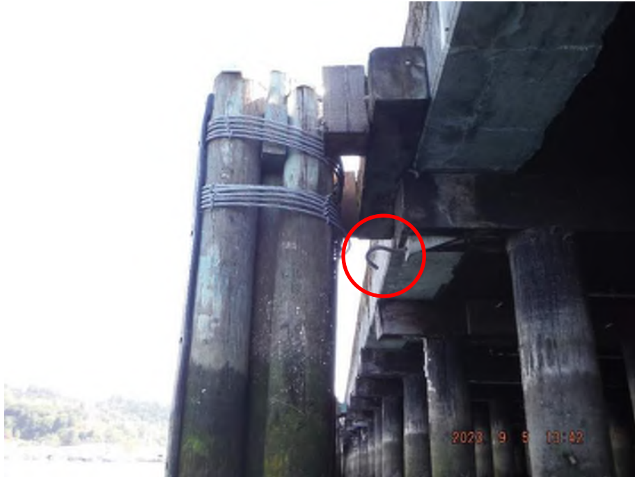
Photo 9 – Fender System Disconnected from Wharf at Bent 21.
