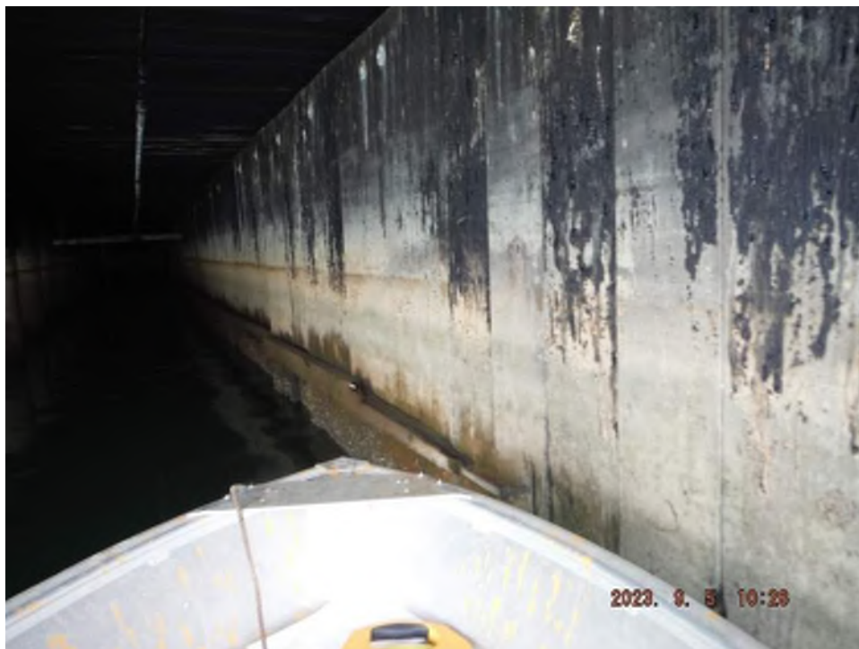
Photo 15 – Typical Above-Water Condition of Firewall.
