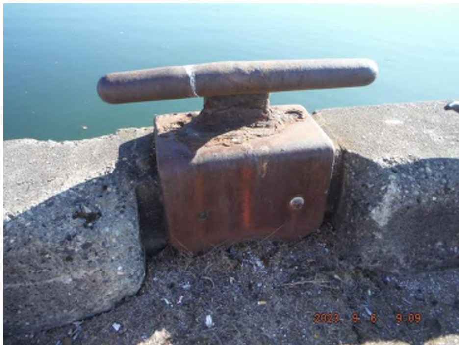
Photo 4 – Cleat with Section Loss at the Neck, Missing Anchor. Surrounding Bullrail Mechanical Spalling at Bent 79.
