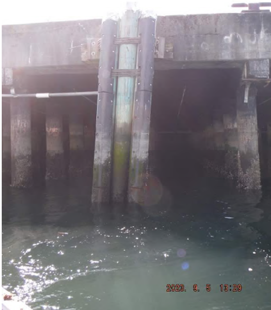
Photo 11 – Fender Piles Out of Plumb and Split Chock at Bent 104.
