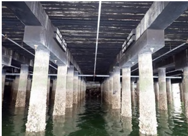
Photo 1. Typical Below-deck Framing
