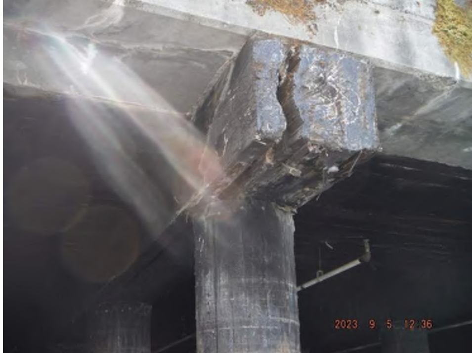
Photo 14 – Major Split in Pile Cap End at Bent 88.
