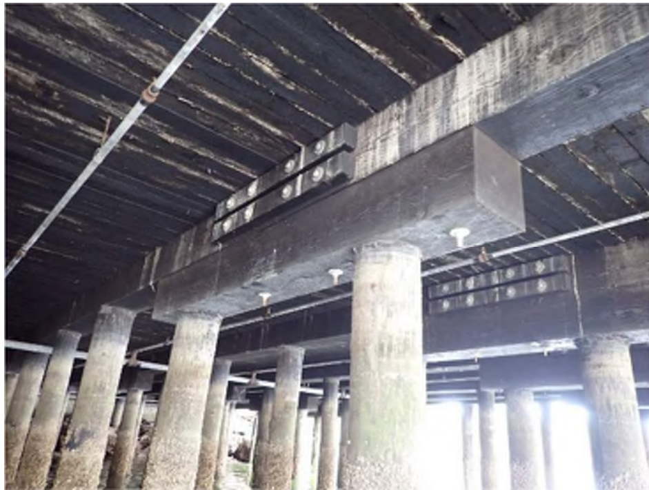
Photo 13 – Typical Pile Cap Splice.
