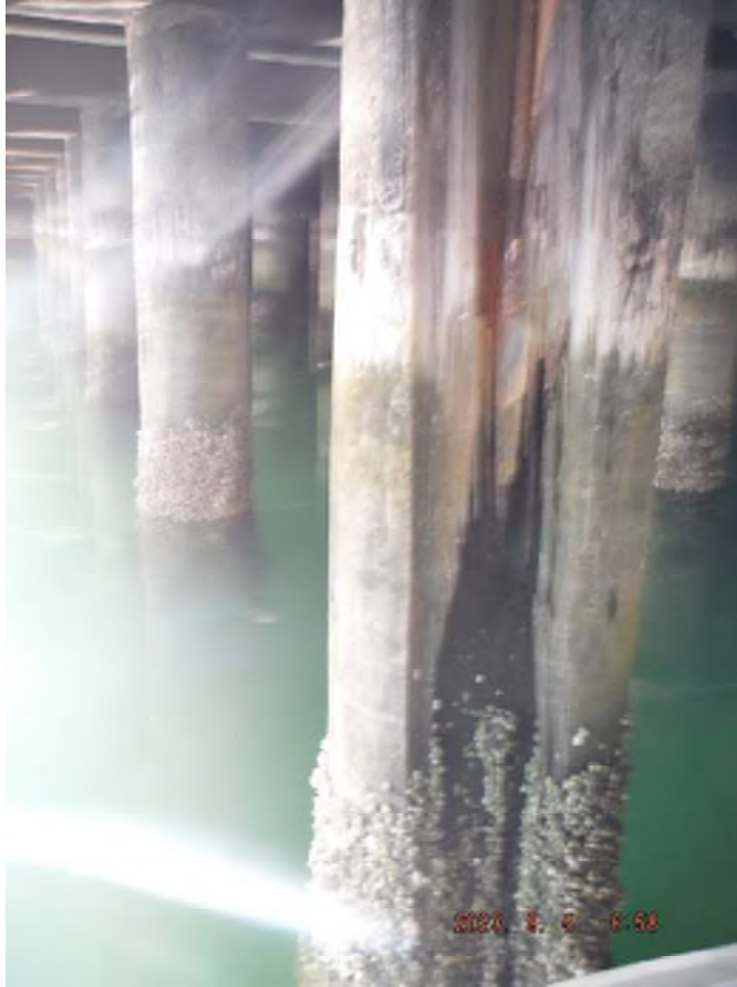
Photo 18 – Pile Cross Section Major Loss at Waterline, Pile 4:B.
