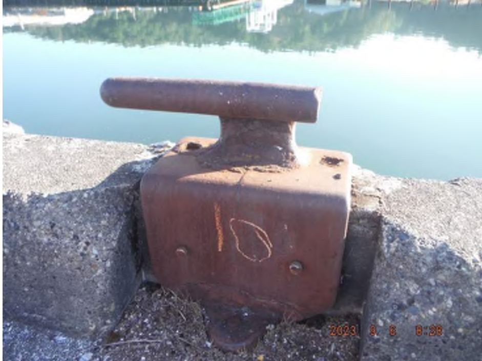
Photo 5 – Cleat with Broken Ear at Bent 10.
