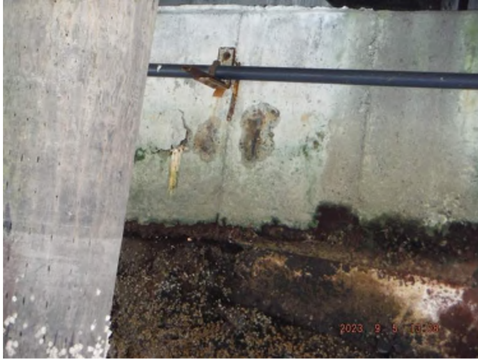
Photo 16 – Open Spalling with Exposed Reinforcement in Bulkhead Pile Cap at Bent 11.
