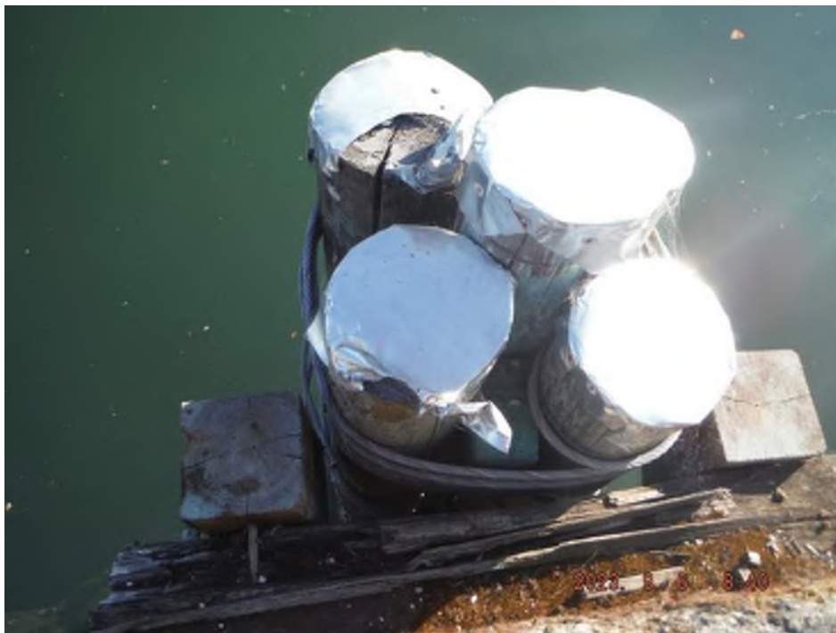
Photo 8 – Split Wale with Exposed Anchor and Rot. Split Pile with Torn Sheet Metal Hats at Bent 34.
