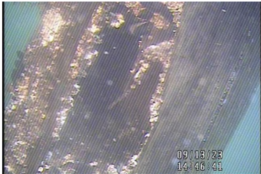
Photo 19 – Cavity in Pile GP-2:A. Severe Section Loss.
