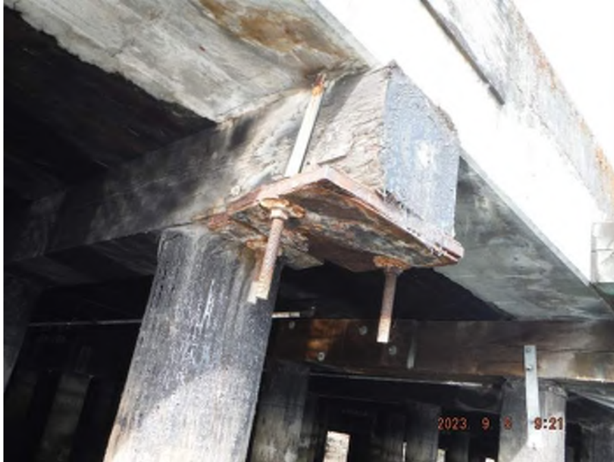
Photo 7 – Moderate Corrosion of Bearing Plate that Anchors the Mooring Fitting at Bent 101.
