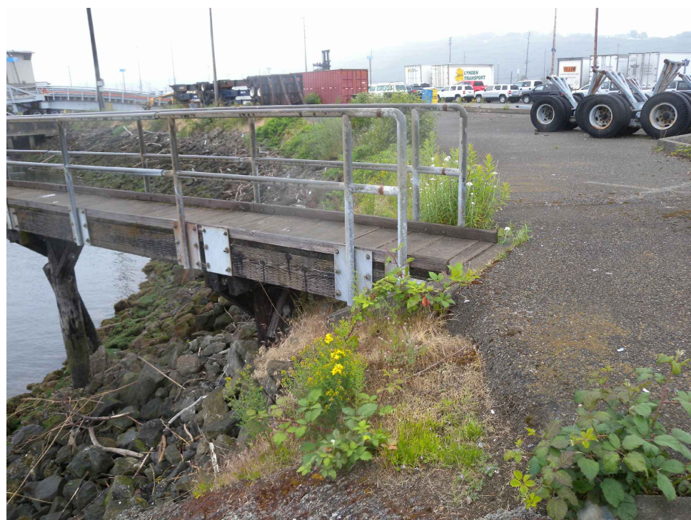
P1 EXISTING CATWALK
