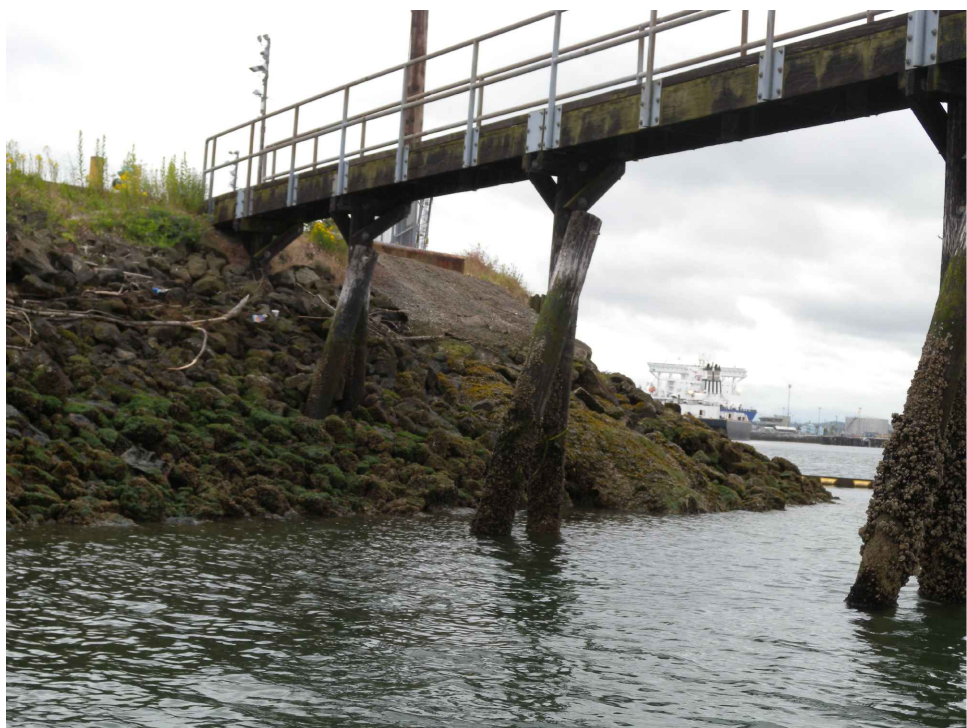
P2 EXISTING PILING
