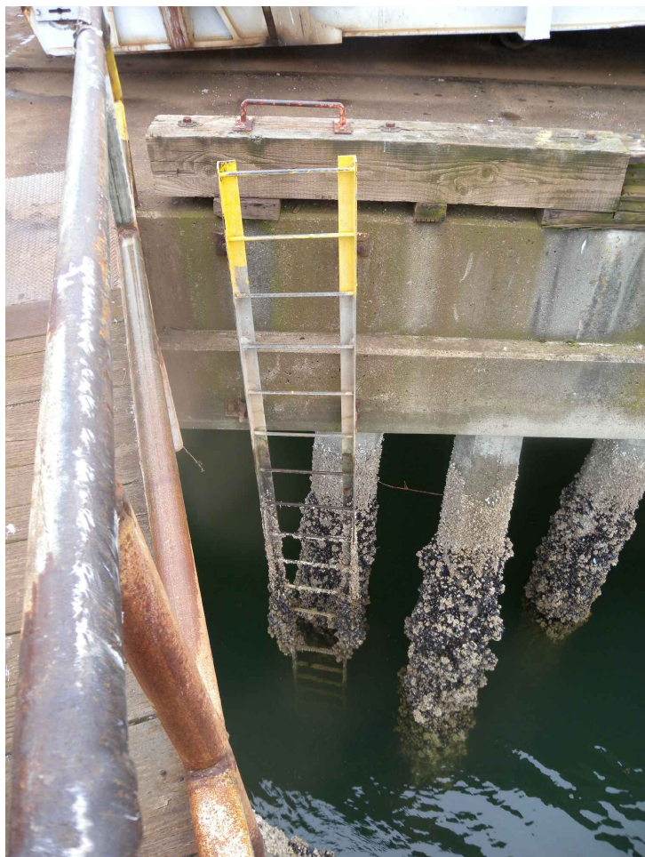
P3 EXISTING LADDER
