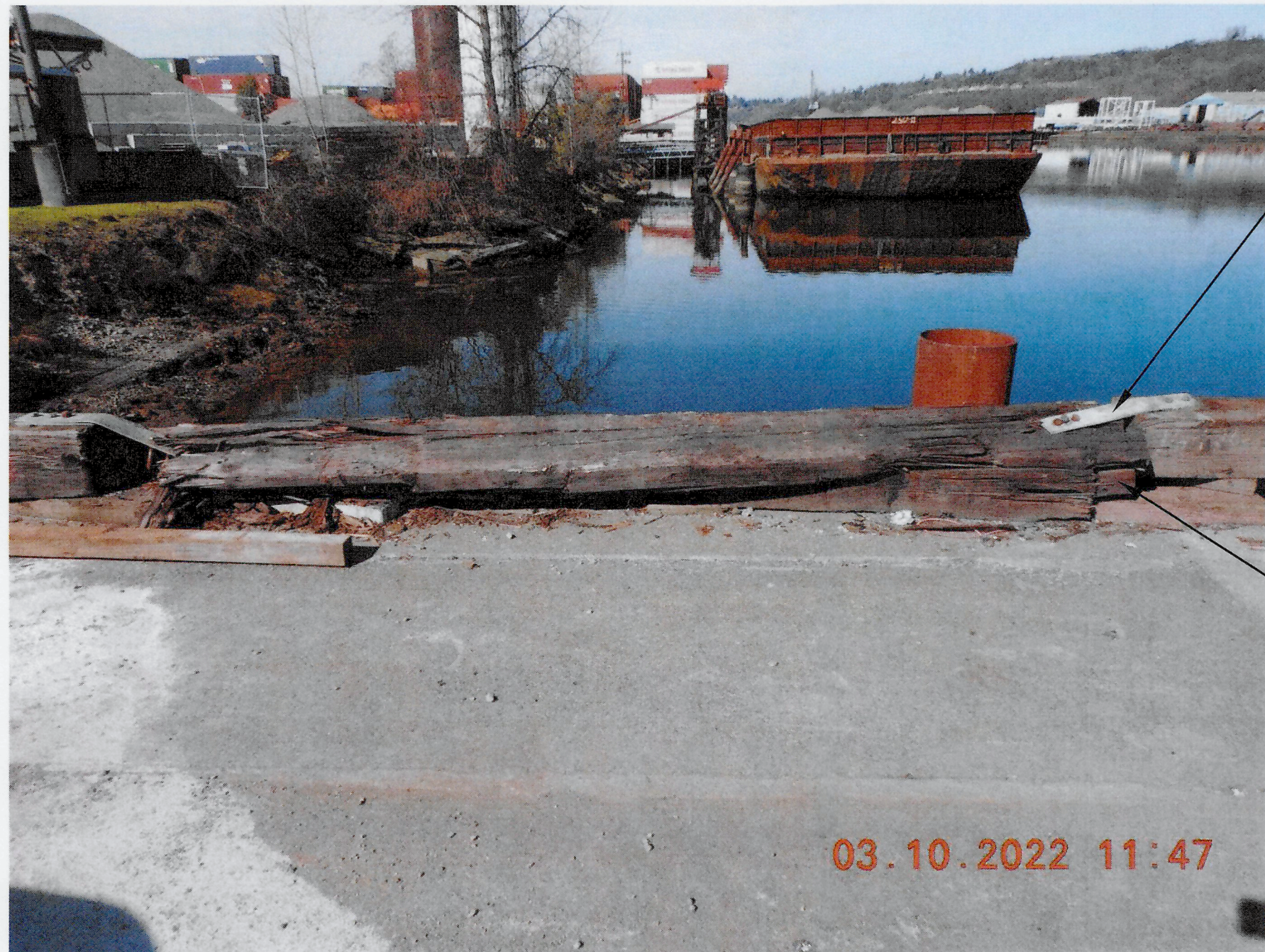
P2 G3 BULLRAIL LOOKING: WEST
