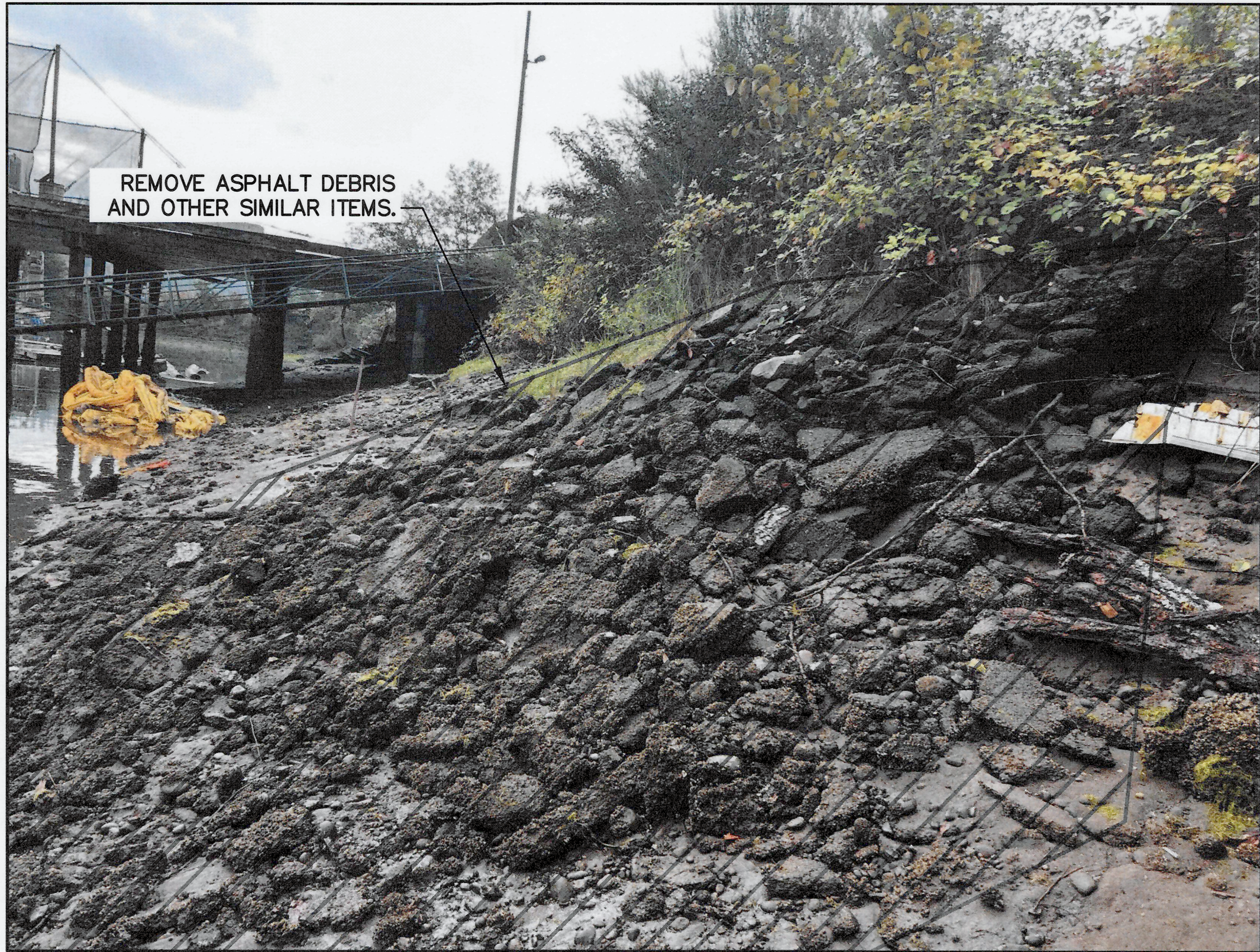
P3 — WEST DEBRIS REMOVAL LOOKING: EAST
