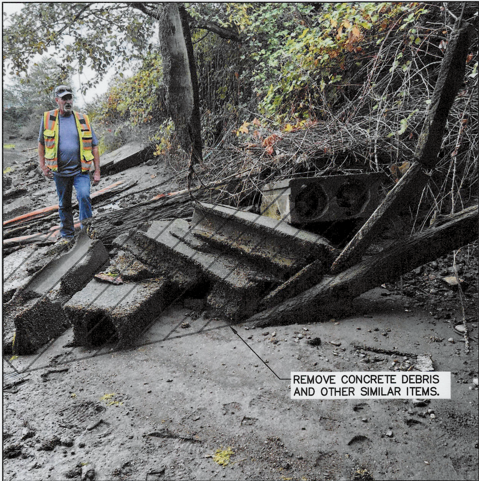
P3 — UNDERDECK DEBRIS REMOVAL LOOKING: SOUTH
