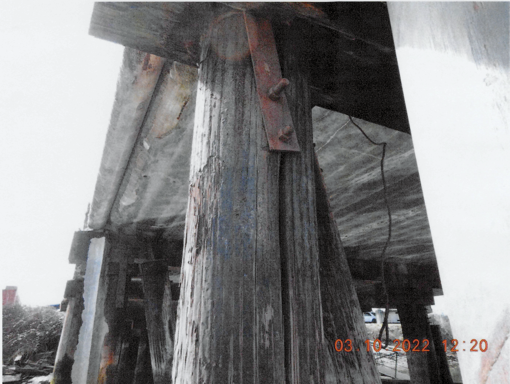
P4 G3 SPLIT PILE LOOKING: SOUTH
