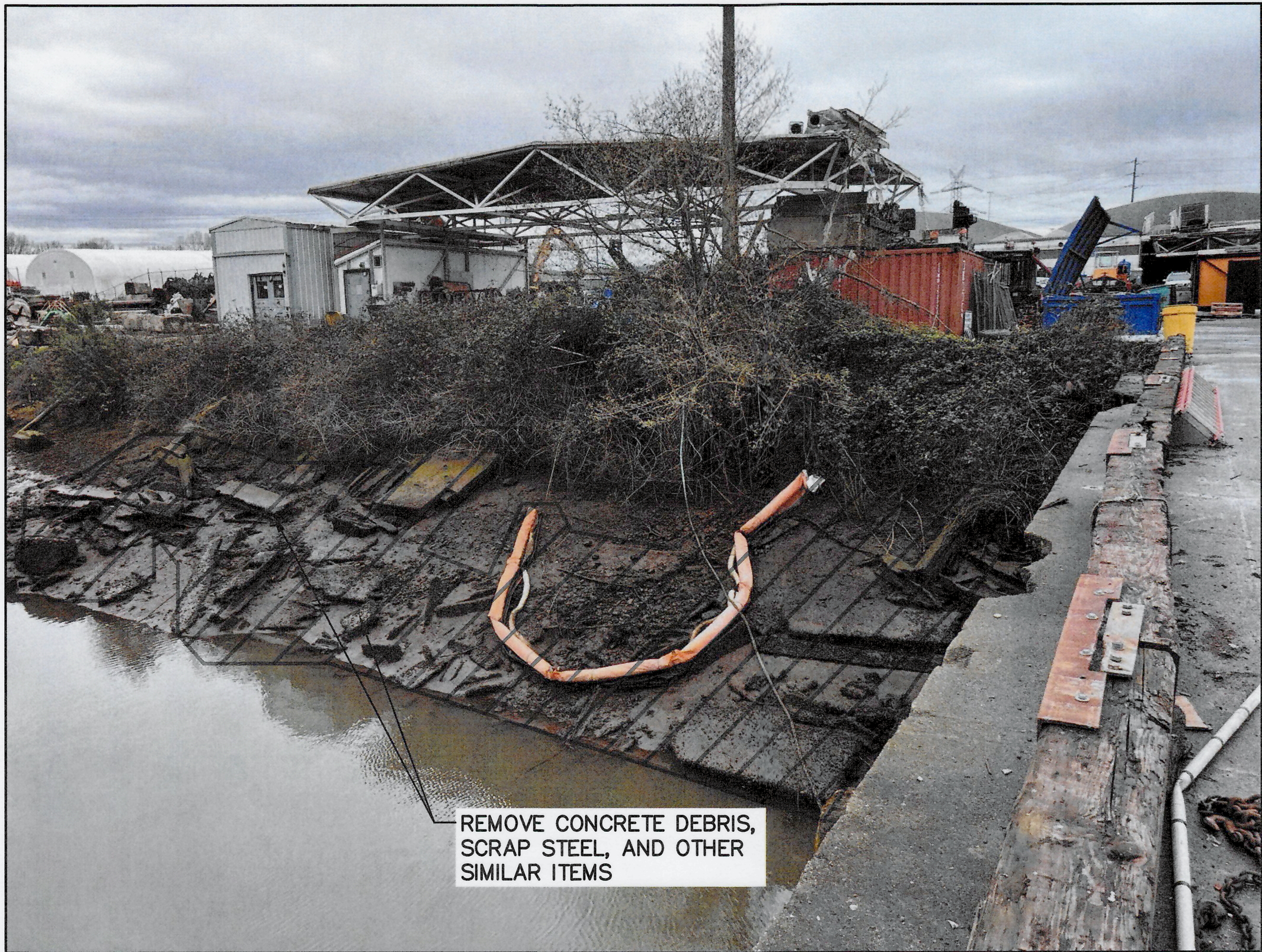
P2 — EAST SHORELINE DEBRIS REMOVAL LOOKING: SOUTH
