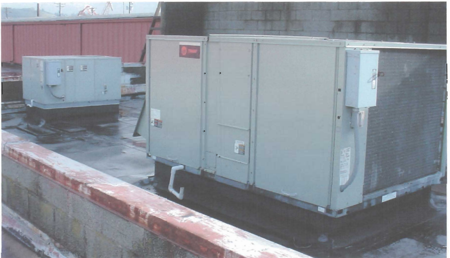
New roof-mounted air handling unit in place.
