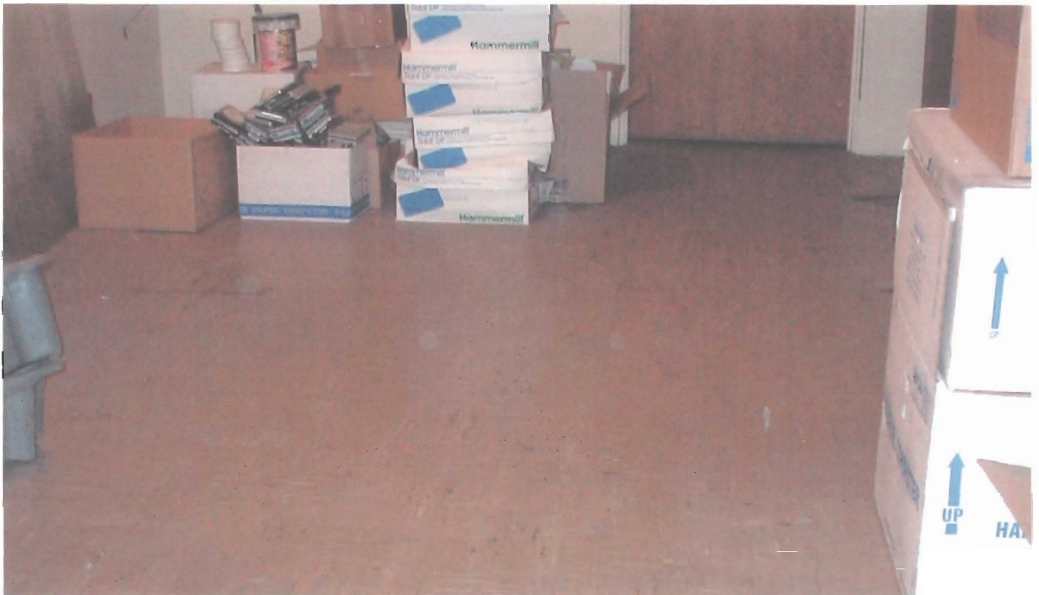
Typical office floor covering - 9-inch VAT.
