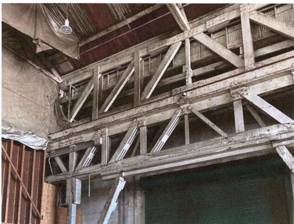
12 (E) GIRDER TRUSS #6 A5.1 NTS
